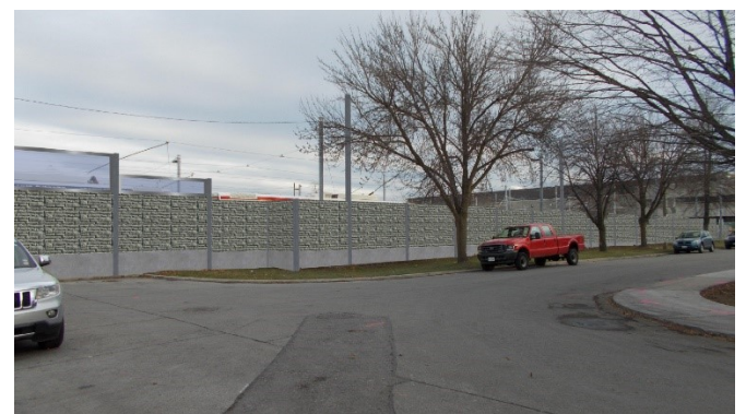
West wall view from Minto Street
